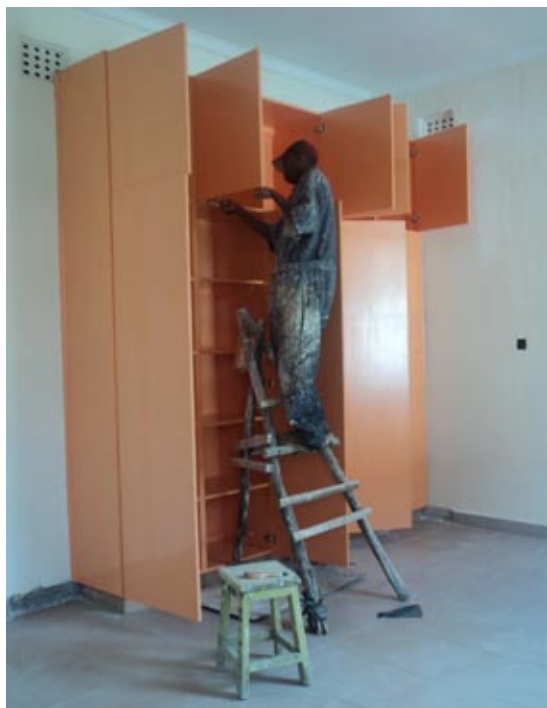
On going renovations in the wards
