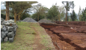
Digging the hospice foundations at Kijabe
